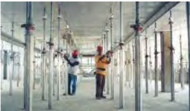
Proper calculations reduce risks when pouring slabs.
