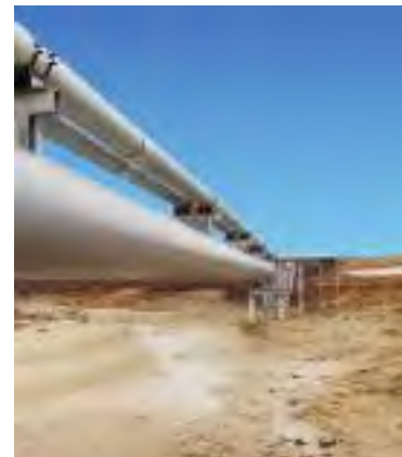
Based on the agreement, 25mn cu/m of gas will be delivered to Sadr, Baghdad and al-Mansouryah power plants through a 270 km pipeline. (Photo: Sergii Ryzhkov)
