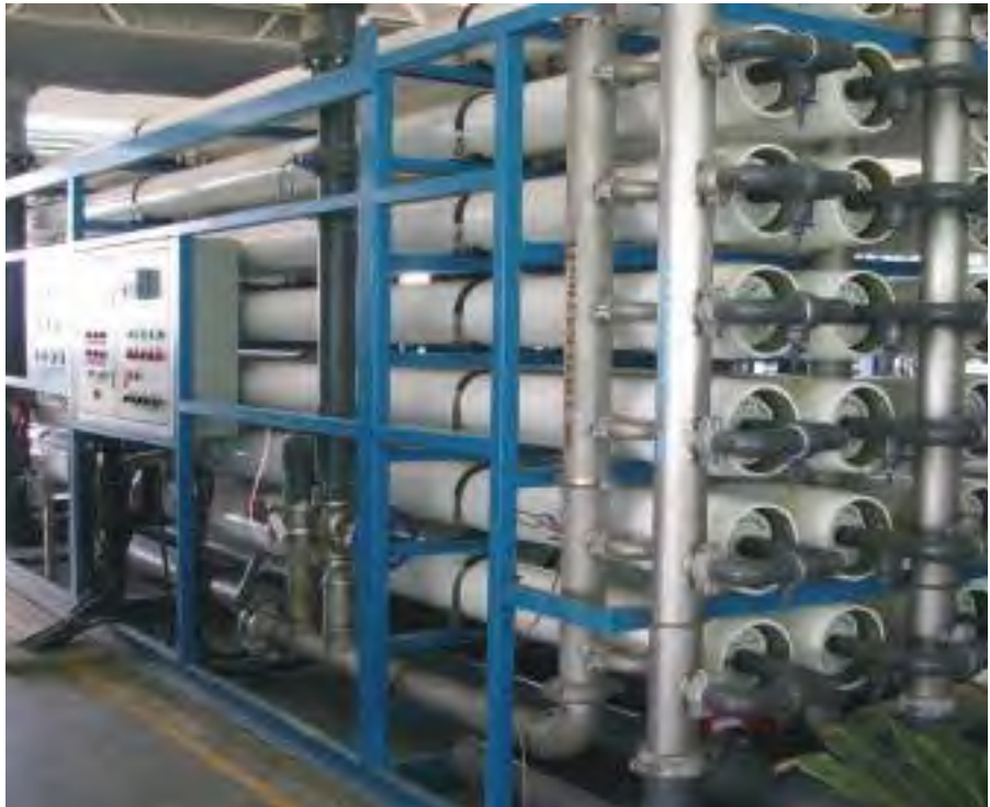
The emphasis in the region is shifting to the less energy intensive reverse osmosis process (Photo: Lee Sean)
