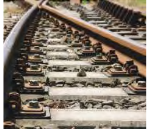
Alstom will carry out major improvements to the Beni Suef-Asyut line in Egypt (Photo: fcl1971)
