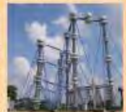
HVDC Generator at UHVRL Hybrid
