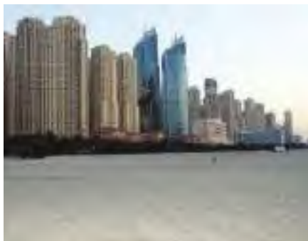
The environment in Middle East is highly corrosive with saline water and airborne salt damaging building near water bodies. (Photo: Imre Solt/Wikimedia Commons)
