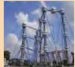
HVDC Generator at UHVRL, Hyderabad
