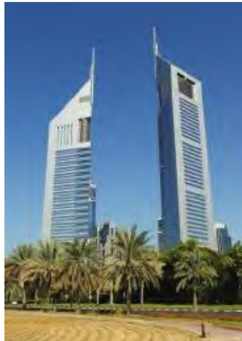
The conversion of the district cooling system at Emirates Towers will result in energy savings of approximately 80 per cent (Photo: Guilhem Vellut)
