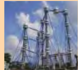
HVDC Generator at UHVRL, Hyderabad
