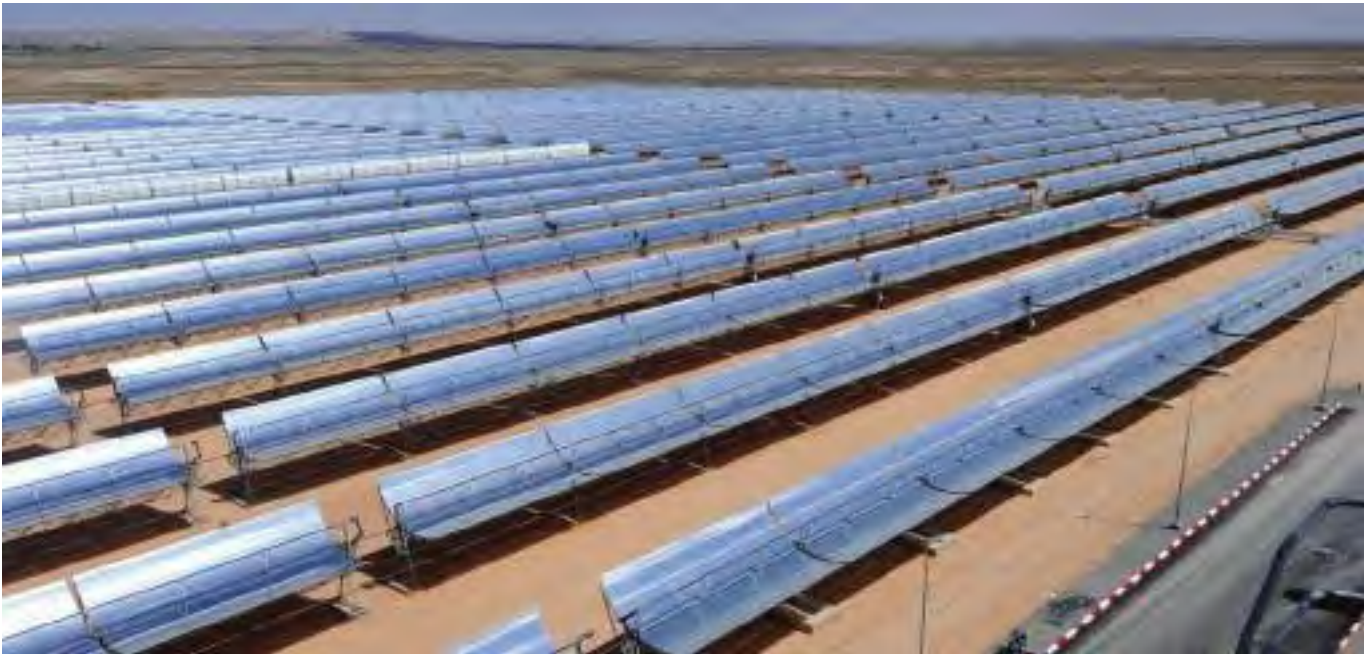
Smart grid solutions are gaining relevance in the Middle East due to the rise in renewable energy projects
