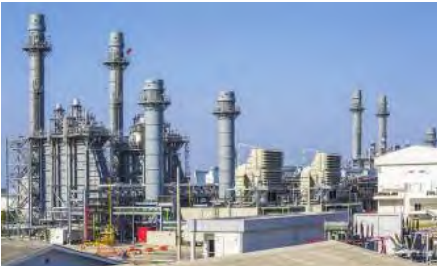
Gas turbine upgrades could help the region meet its growing power needs. (Photo: Photo Smile/Shutterstock)
