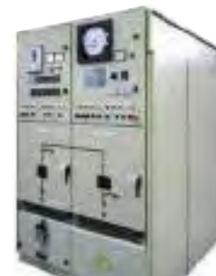
The Normoclad MV switchboard for submersible pumps.
