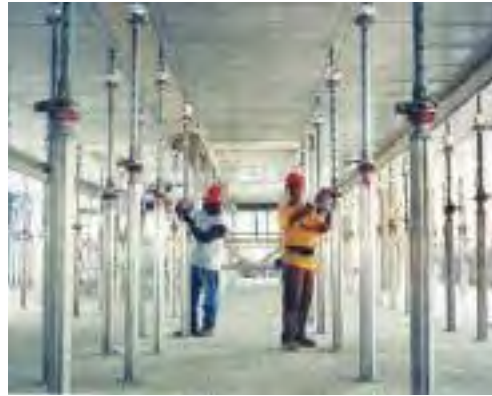
Proper calculations reduce risks when pouring slabs.
