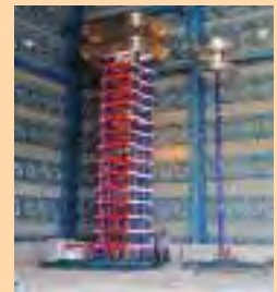
2400kV, 240kJ Impulse Voltage Generator
