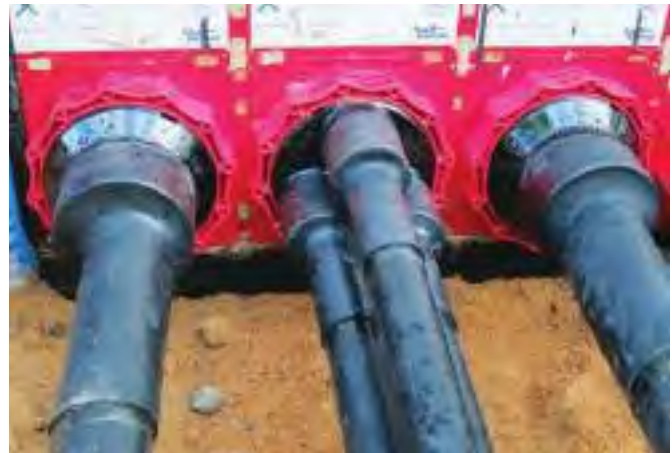
Image 1: The range of system covers includes those with sockets for sealing the cable using a hot or cold shrinking process.
