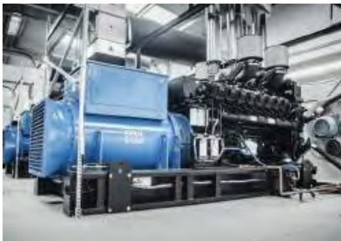
Inside view of the power plant with its four generating sets. The new port will be operational from June 2019 and, in future, the backup power plant may be extended to include 10 generators, if necessary.
