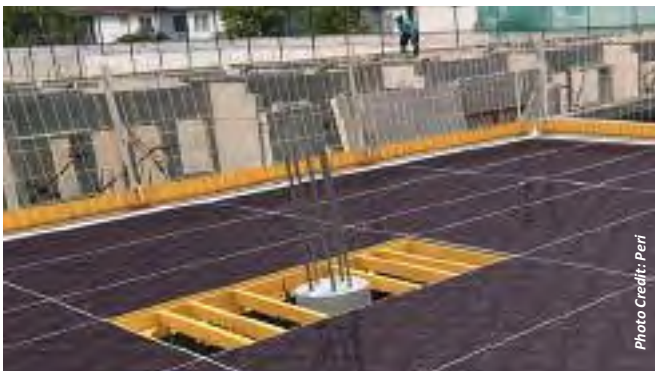
Additional system components such as column frames and adjustment beams make it safe and easy to marry up mating surfaces.
