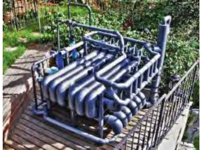
The patented Biopipe system uses a simple process to treat wastewater inside a pipe lined with live bacteria. (Photo: Biopipe)
