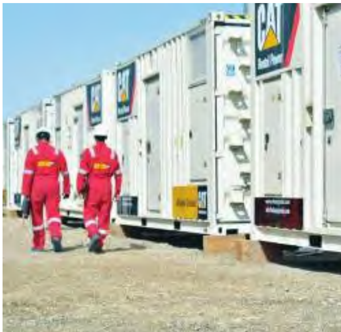
Hiring temporary power generation plants could offer a number of advantage to utility companies
