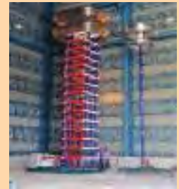
2400kV, 240kJ Impulse Voltage Generator
