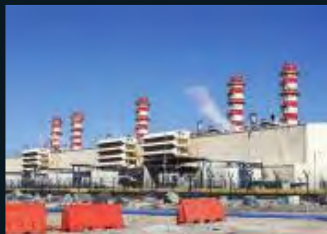
The third phase of the project will start by October 2015. (Photo: Philip Lange/Shutterstock)
