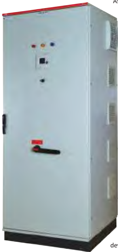
The capacitor bank meets IEC 61439 and IEC 61921 standards.
