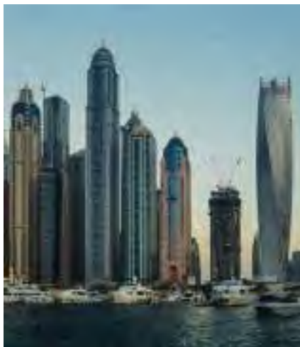
Dubai has been plagued by fire incidents in high-rise buildings. (Photo: Bir/Pixabay)
