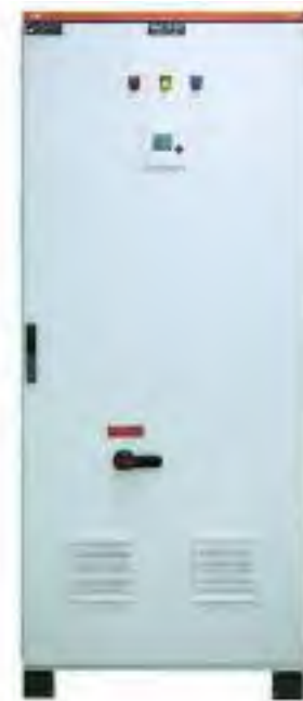
The average lifespan of a capacitor bank is 100,000 working hours.
