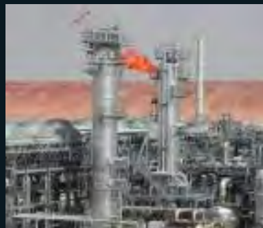
Al Taweelah Alumina is a greenfield refinery project in Khalifa Industrial Zone Abu Dhabi. (Photo: Al-Futtaim)
