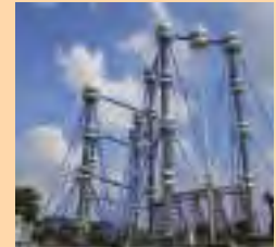
HVDC Generator at UHVRL, Hyderabad
