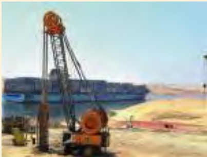
The twin-tube Ismailia road tunnel is scheduled for completion in 2018. (Photo: Bauer)
