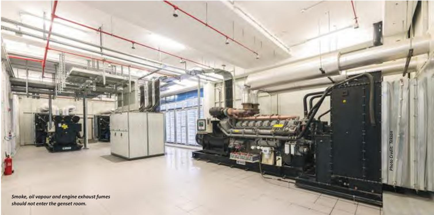
*Smoke, oil vapour and engine exhaust fumes should not enter the genset room.*
