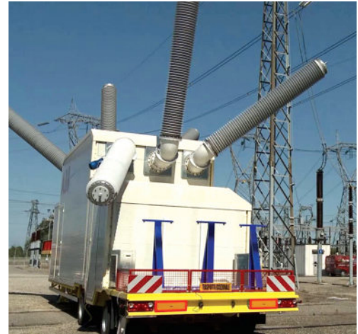
Photo Credit - Hitachi ABB Power Grids
