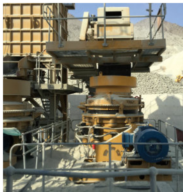
The Trio TP360 cone crusher installed at an operation in Oman.
