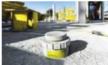
Concremote determines the optimum time for stripping the formwork, increasing productivity. (Photo: Doka)
