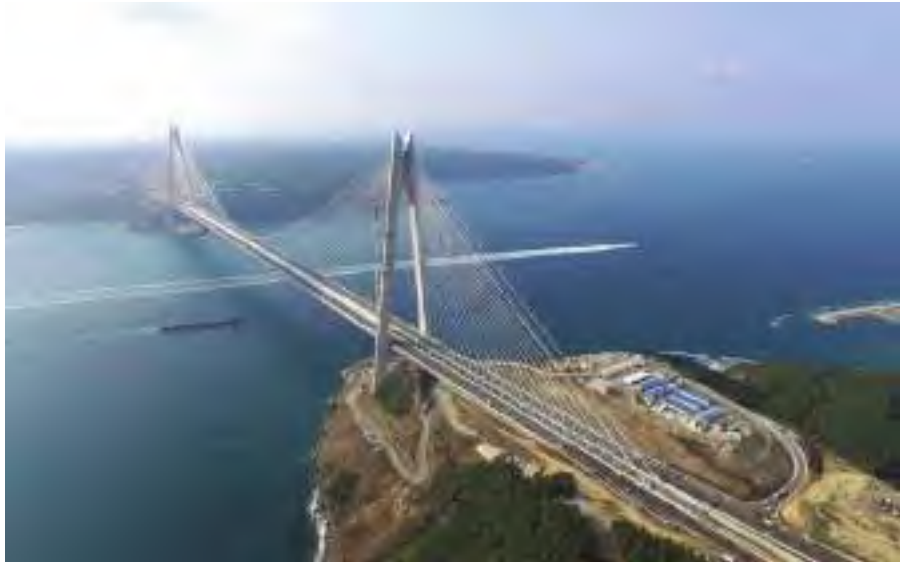
FG Wilson Turkey has installed four 605kVA generator sets to power the bridge's towers, road lighting, tower escalators, service pumps, dehumidification units and architectural lighting. (Photo: FG Wilson)
