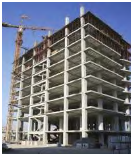
Construction projects to the value of round US$600bn are underway in the kingdom. (Photo: Salem Alfaraih/Shutterstock)
