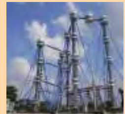
HVDC Generator at UHVRL, Hyderabad
