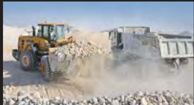
The L958F is responsible for loading the wadi stone (hard limestone pebbles that measure up to 30cm in circumference) into tipper trucks for delivery to the site's crusher hoppers.
