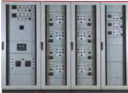
Powertech Switchgear Industries has supplied low-voltage switchgear and panel boards to a number of projects in markets throughout the Middle East
