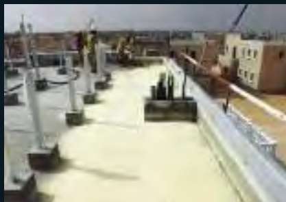
The Solstice LBA is being applied to villa roofs in Al Ain.
