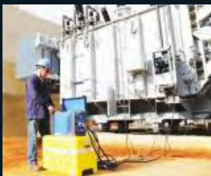
The integrated three sources and the simple wiring concept speed up and simplify power transformer testing.
