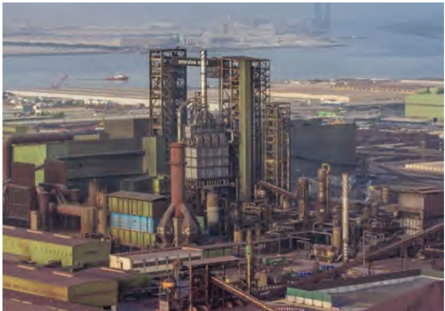
Photo Credit: Emirates Steel
