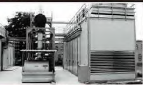
Bio Oil 2MW Power Plant - Italy
