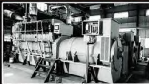
Yoboki-Lac Assal HFO 4.8MW Power Plant - Djibouti
