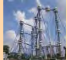
HVDC Generator at UHVRL, Hyderabad
