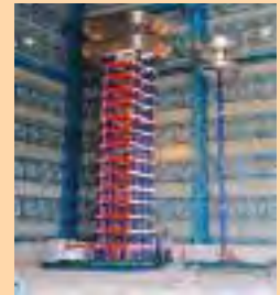
2400kV, 240kJ Impulse Voltage Generator
