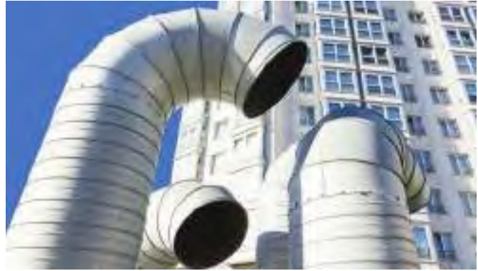
Saudi Arabia will be among the fastest growing markets for HVAC equipment between 2015-2020, according to The Freedonia Group. (Photo: Gena Fotografo)
