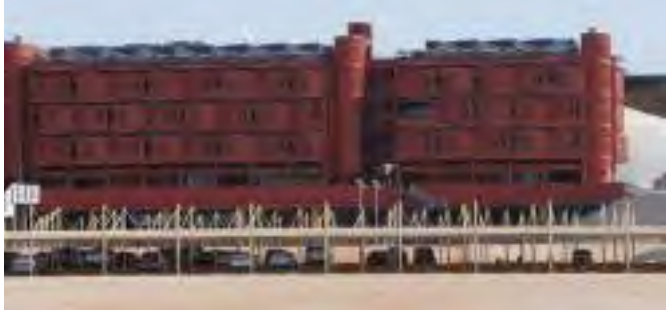
A number of projects throughout the GCC, such as Masdar City in Abu Dhabi, have helped raise the profile of 'green building' techniques. (Photo: Masdar)
