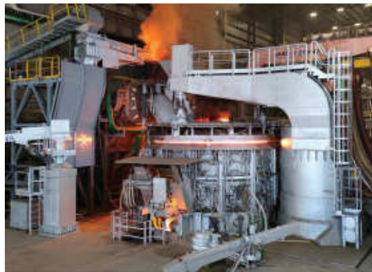
SMS CONDOOR in operation at the Hidd Industrial area.
