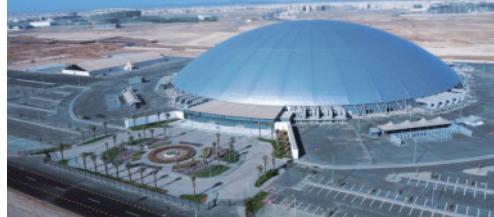
Aerial view of Jeddah Superdome venue.
