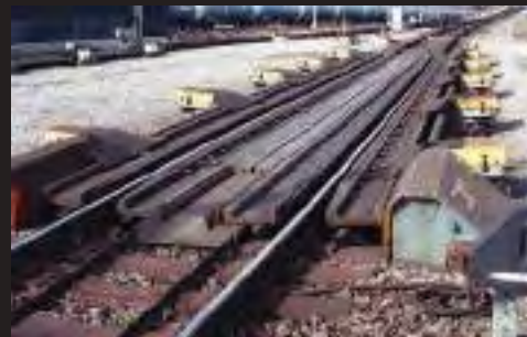
Huawei's GSM-R technology allows for railway signalling and operational communication even when trains are at high speeds
