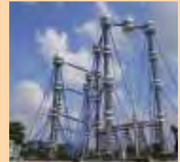
HVDC Generator at UHVRL, Hyderabad
