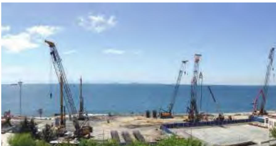
The 5.4 km-long twin-deck Eurasia tunnel will connect the European and Asian parts of Istanbul
