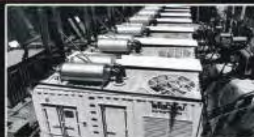
High Voltage 6.3MW Power Plant - Thailand
