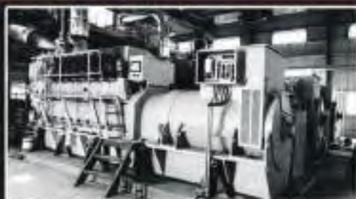
Yobeki-Lac Assal HFO 4.3MW Power Plant - Djibouti
