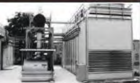
Bio Oil 2MW Power Plant - Italy
