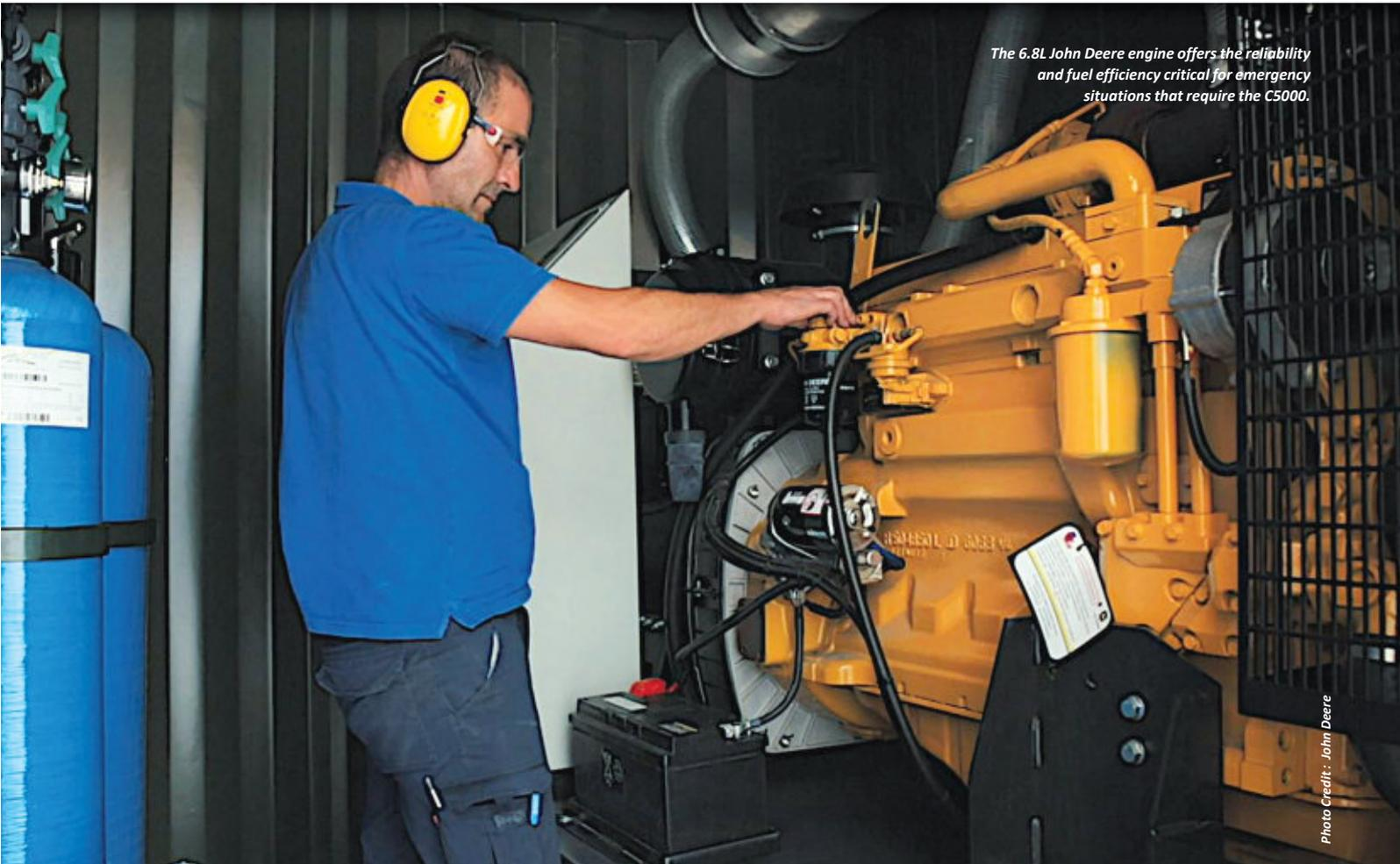
*The 6.8L John Deere engine offers the reliability and fuel efficiency critical for emergency situations that require the C5000.*
