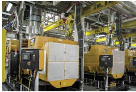
Al-Bahar and Caterpillar teams worked together with Lamprell right from the inception stage of the project to design the final power solution needed for the rigs.
