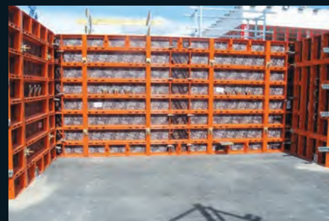
LOGO.3 wall formwork system can withstand a high maximum fresh concrete pressure.
