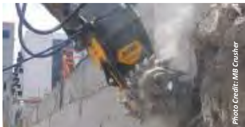
Drum cutter MB-R800 on Caterpillar excavator.
